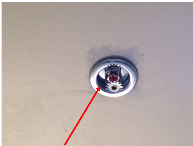
Semi-recessed head with less than 1/2" clearance below the ceiling surface
