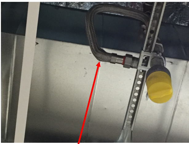
Crimped the hose during installation to achieve center tile
