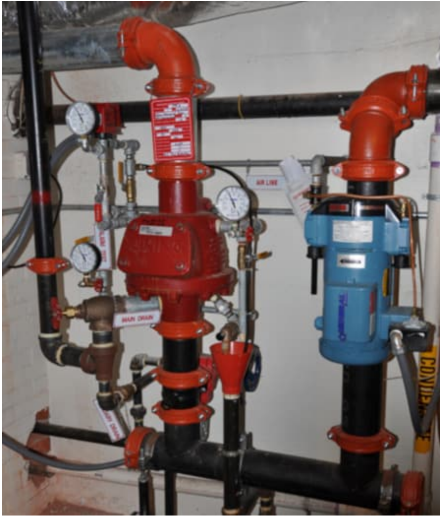
A riser-mounted air compressor (right) and a dry pipe valve (left) in a dry sprinkler system. Source: A.L. Fire Protection
